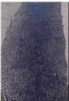
Repairs prior to surface treatment
