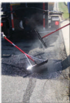
Patch pavement deterioration & pothole repair
