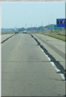
Repair longitudinal & shoulder joints
